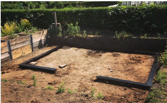
1) The perimeter foundation is positioned, leveled and concreted into position.
