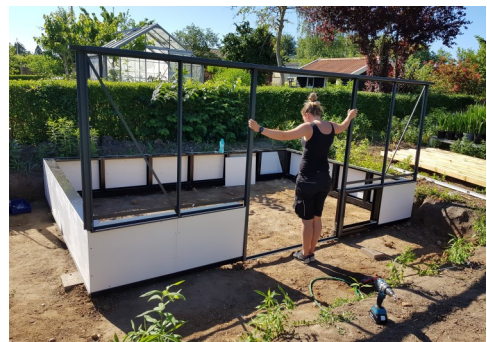
The greenhouse is then assembled on the dwarf wall.
